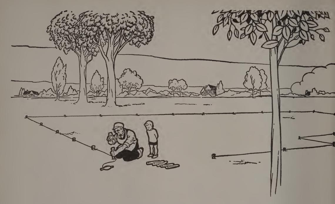
Chips marked the size of the house on the ground. He pounded a number of stakes into the ground and then connected them with a heavy string. Now he knew just where to build the house.
